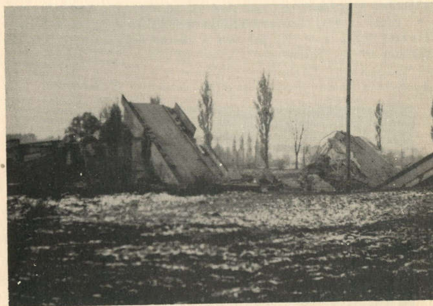
Blown-up bridge across the Isar River at Dingolfing, Germany.
