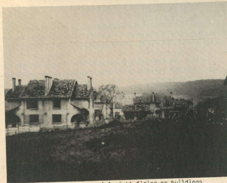
Effect of our special night firing on buildings in barracks area occupied by German troops
