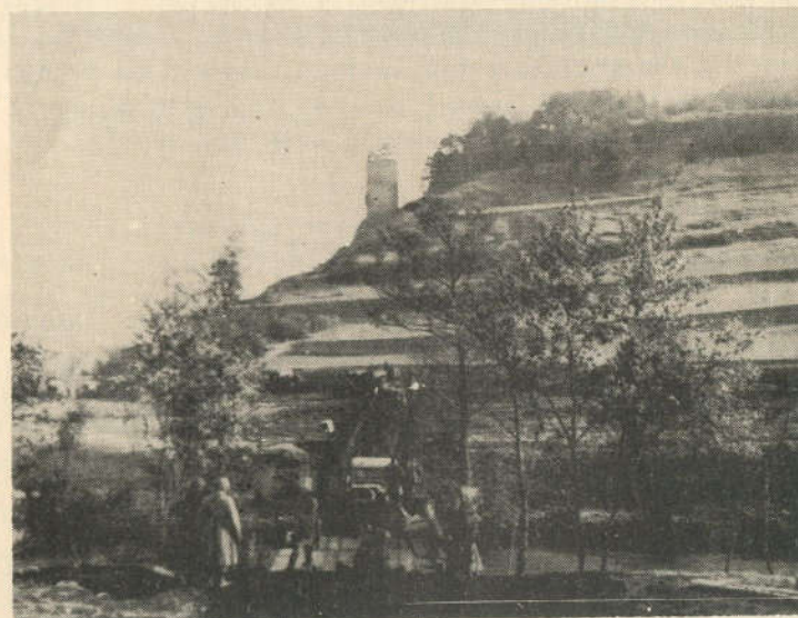
The bridge built for light cavalry scout cars, but we put our 13 ton Howitzers and 13 ton tractors over it.
