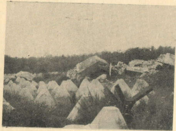
Dragon's Teeth in Siegfried defenses. Note demolished reinforced concrete machine gun pill-box in background
